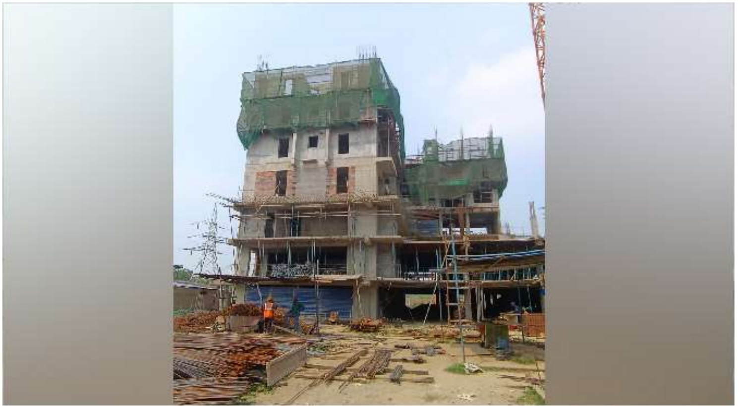
TOWER-1, 7TH FLOOR LEVEL SLAB WORK IN PROGRESS
